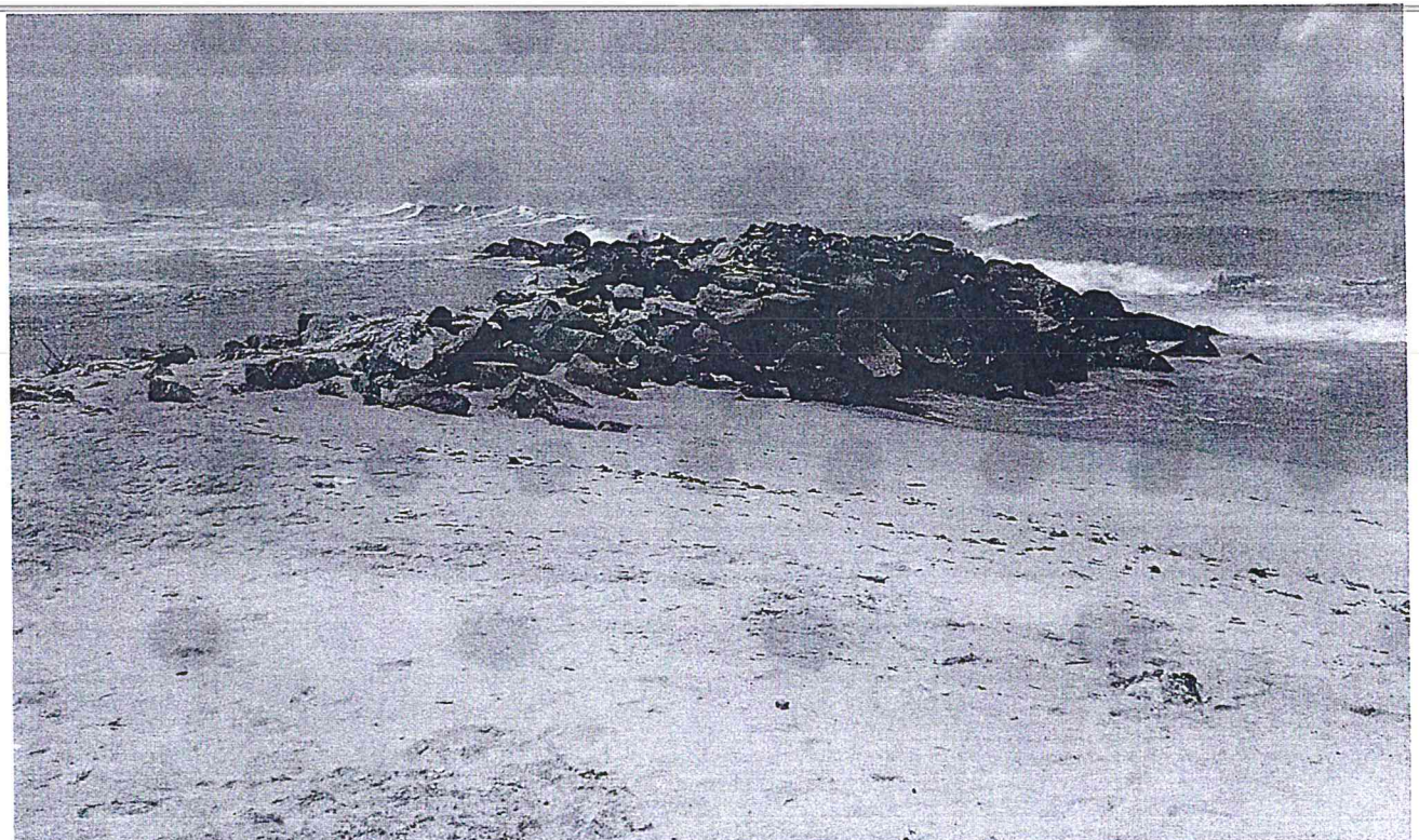
Fig. 7: Erection of Sea defense as a result of excessive sand winning
